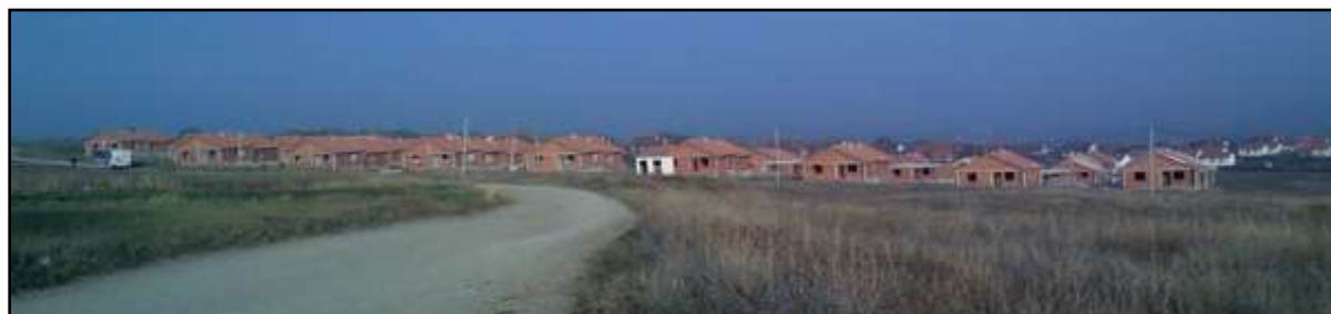
Incomplete Secondary Return Site in Novi Badovac
