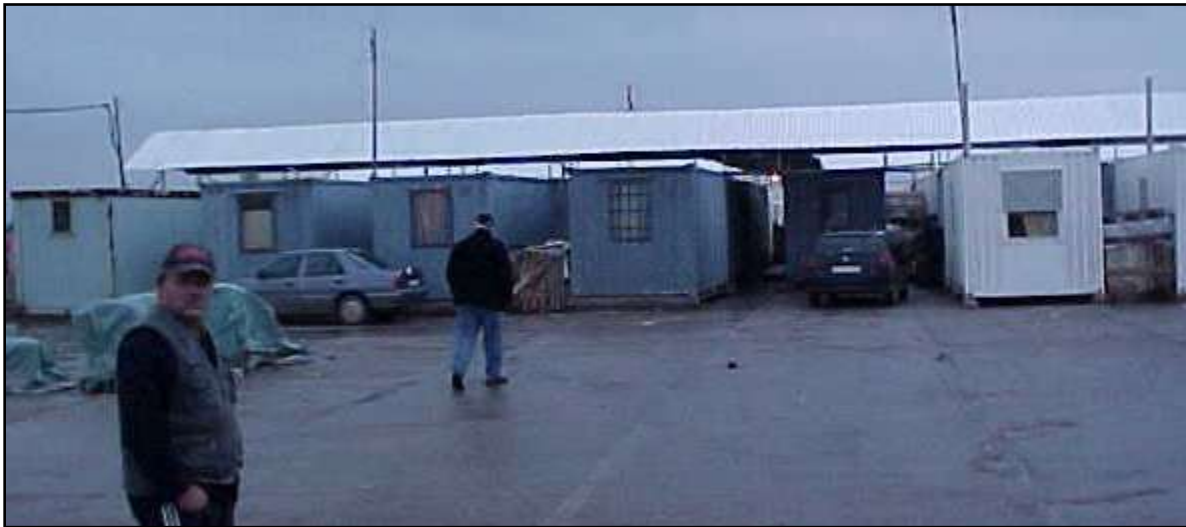
Container Village for IDPs in Gracanica from 2004 - present, is it adequate housing?
